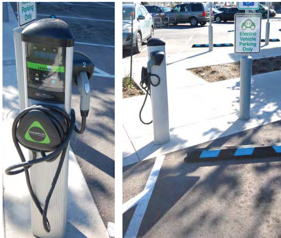
Electric Car Charging Station and Designated Parking
