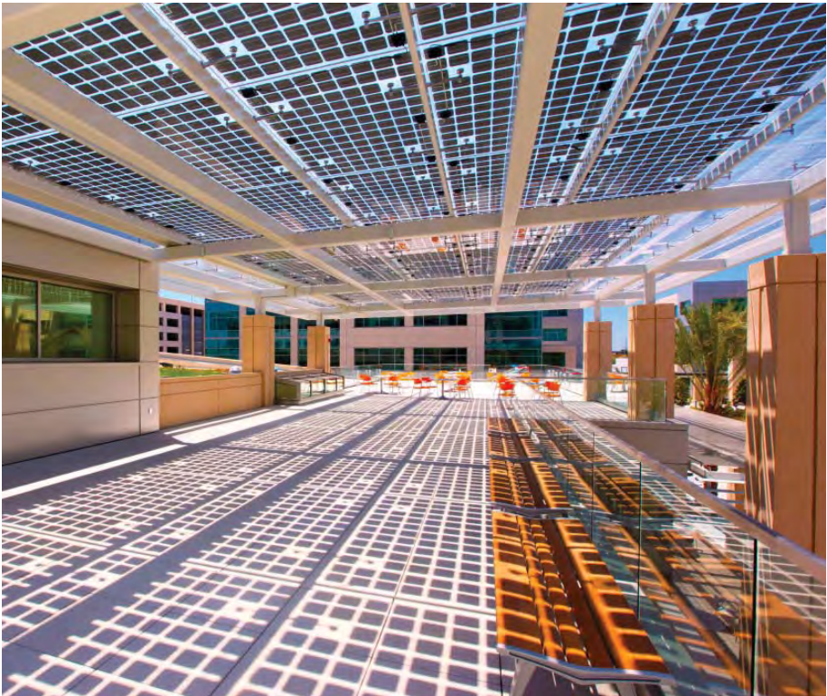
Building Integrated Photovoltaic (BIPV)
